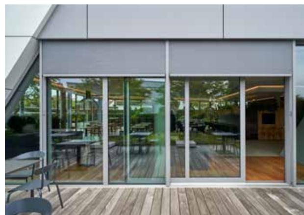
heroal VS Z with the heroal S 77 SL lifting-sliding door system
